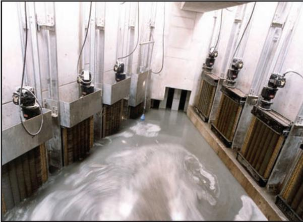
*Nine Discreens installed in a stormwater pumping station*
