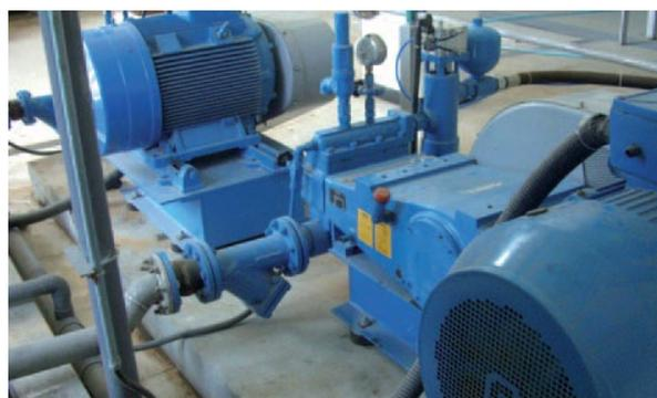
Electro-pneumatically actuated ABEL 3/2- way bypass valve
