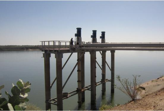
Vertical line-shaft pumps enable considerable savings to be achieved in the construction of pumping stations.
