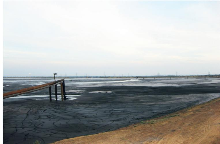
Ash dyke - an ABEL HMQ pump conveys the ash slurry with 65% concentration to this spot 7.5 km away - with such little water content the dry ash solidifies in 3 to 5 hours
